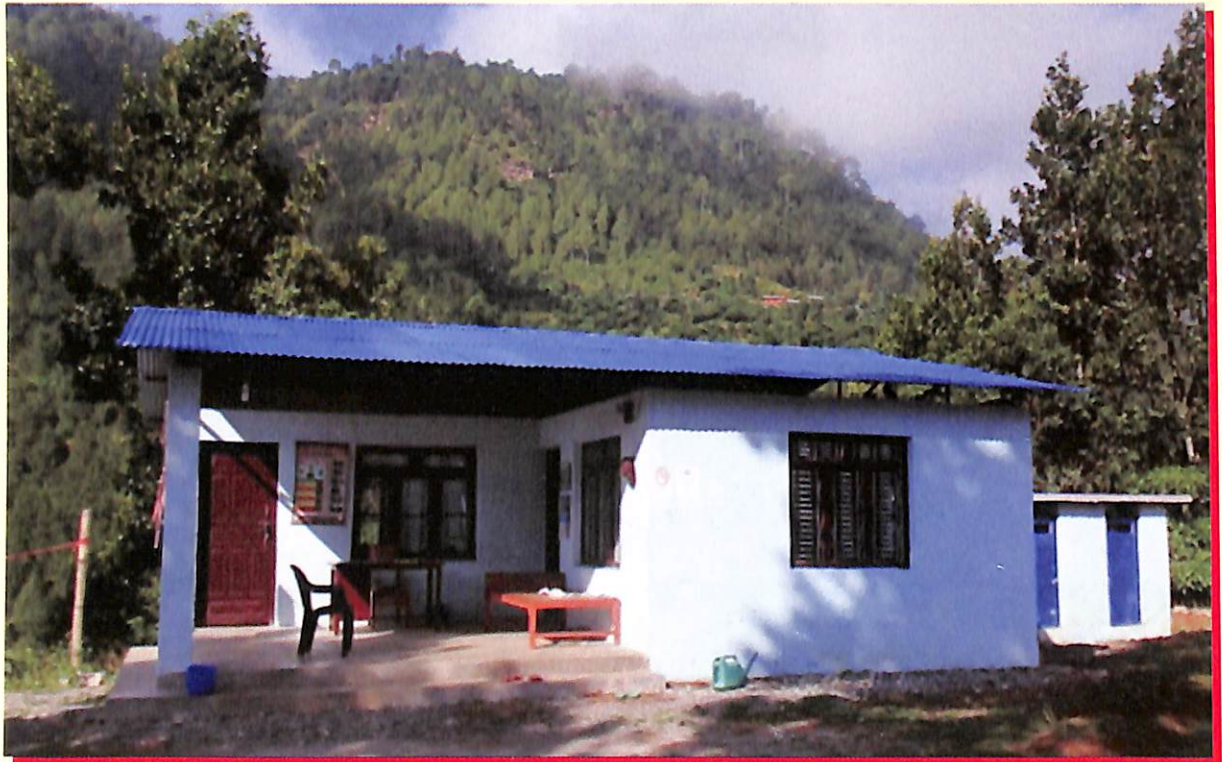
Shed/Watchman Building, CRP Gulmi
